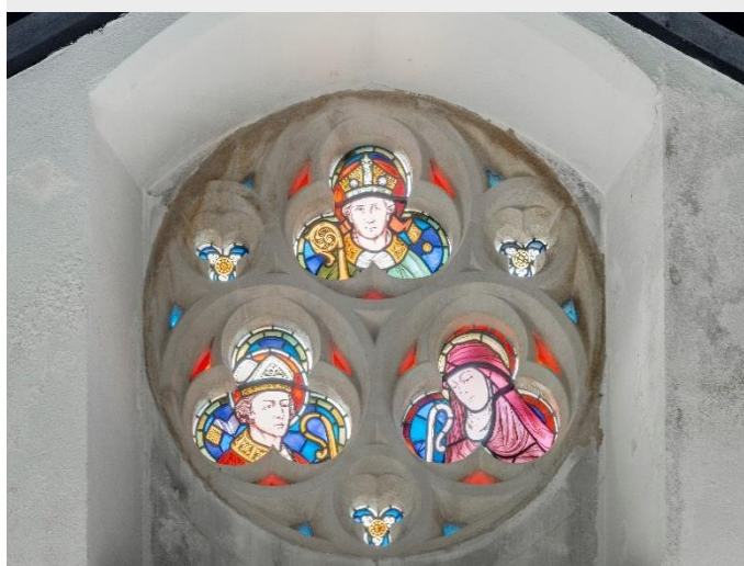
Window Repairs. Photo credit: Purcell UK Architects.
